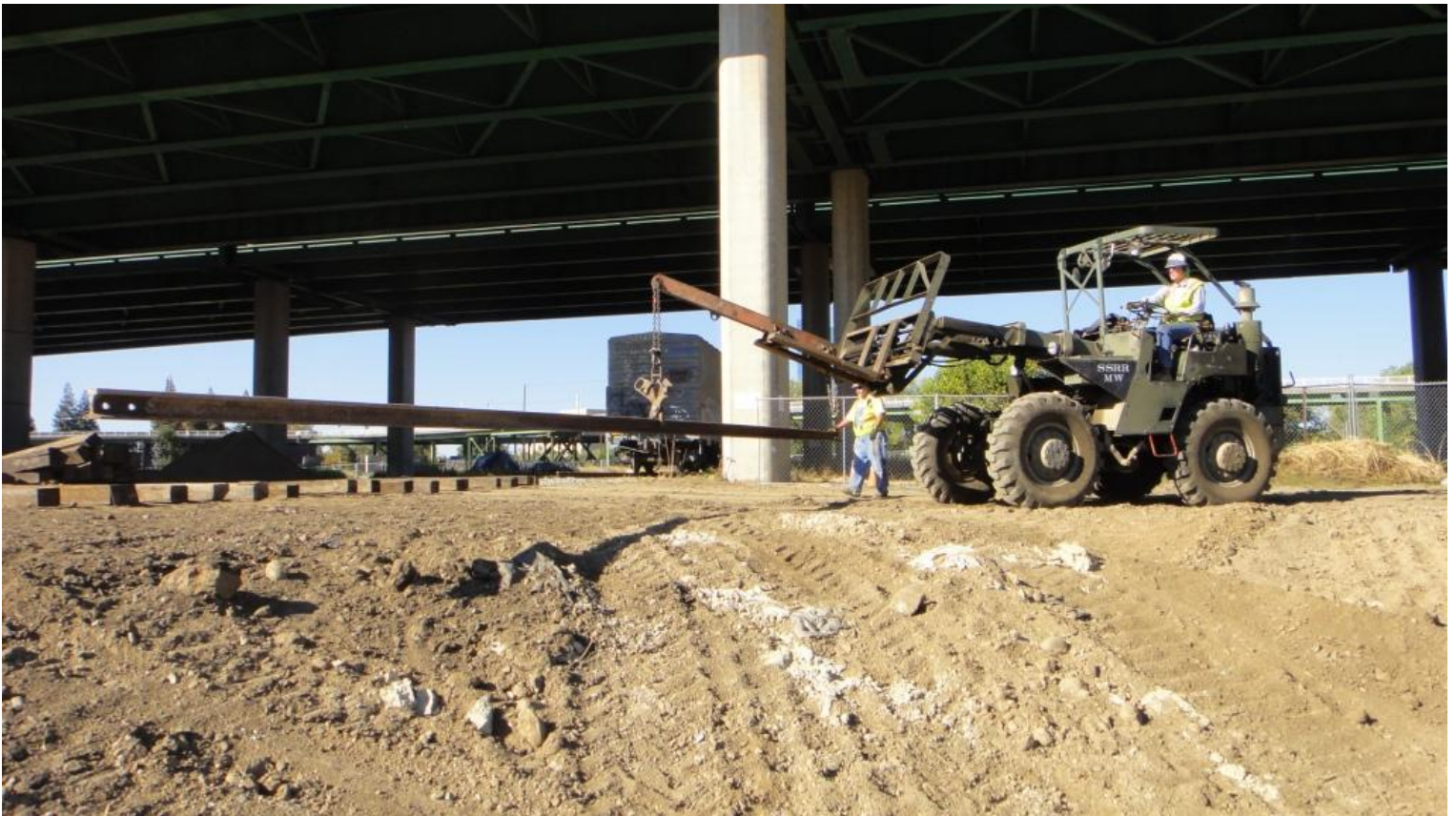
Steve nimbly maneuvers through the Rail Yards carrying a 39-foot ton-and-a-half stick of rail which Mike T. guides
