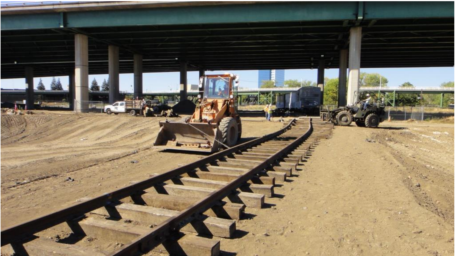
Mike H. in the loader and Steve on Big Green start curving the track
