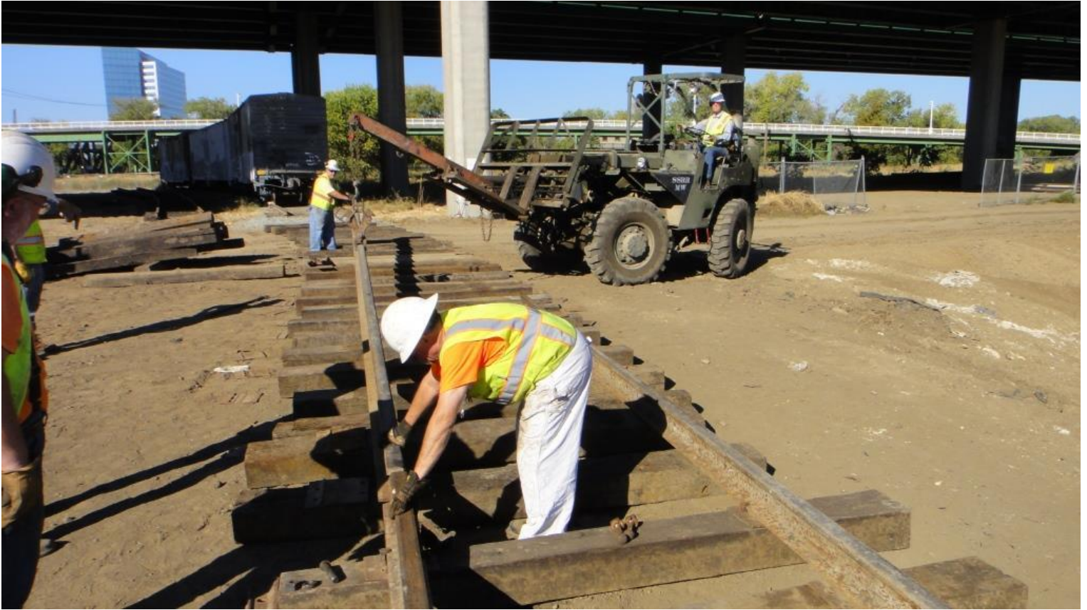
Mike H. guides the east end of the rail to match up with the track that's already in place
