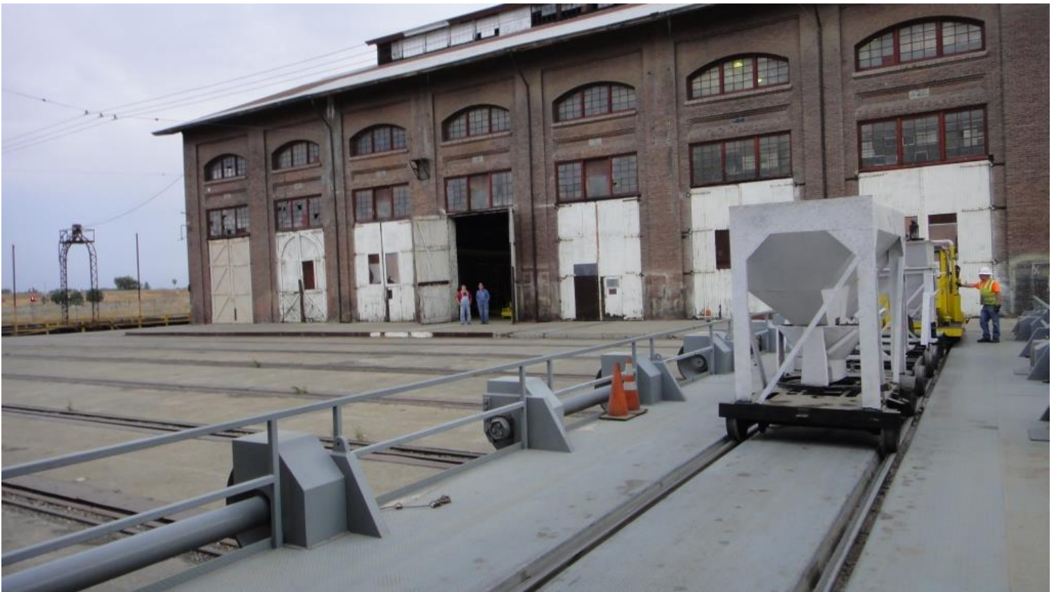
Pat and Cliff await the arrival of the hoppers at Bay 4 of the Erecting Shop
