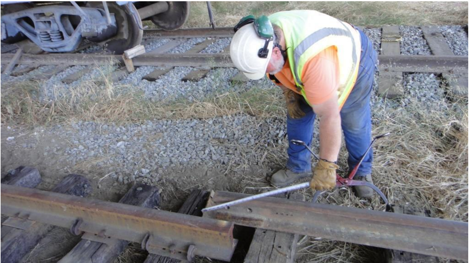
Missed it by that much... Not bad, really, as Frank measures the distance the track laid last week (spotted by eye-ball) and the new track
