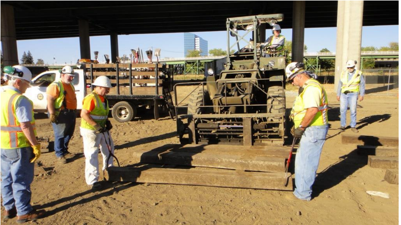
Mike H. and Mike F. begin placing ties for the remaining section of the Firing Line storage track
