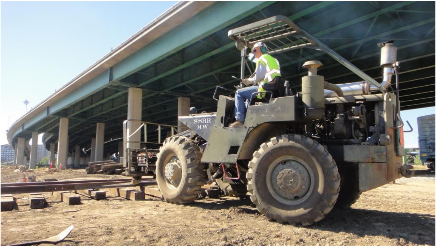
Steve, on Big Green, pushes the track from one end...
