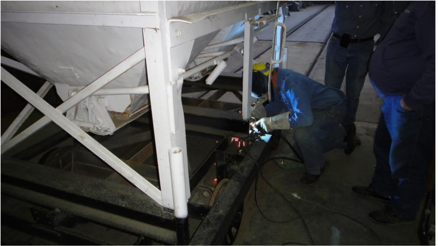
Cliff welds the brake handle back on the center dump hopper car
