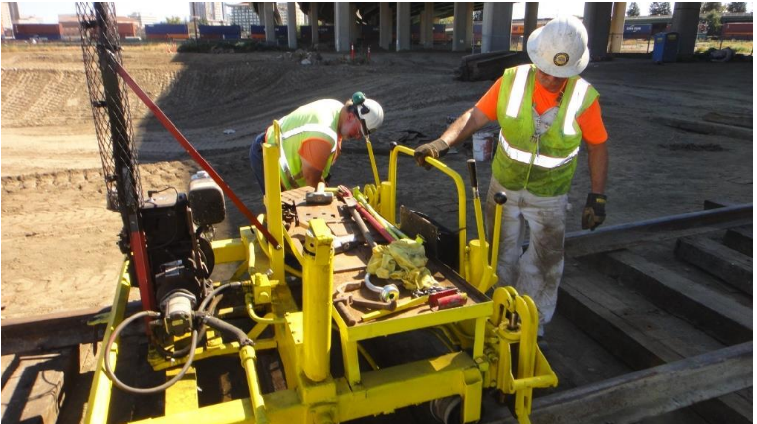
Frank and Mike H. use the rail-lifter to line ties and place tie-plates
