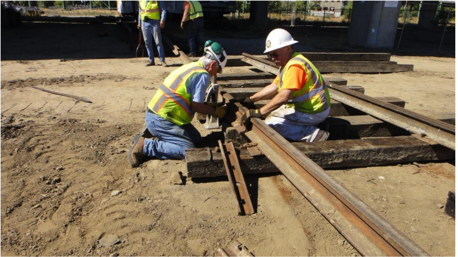
Mike W. and Mike H. connect the two rails with joint bars
