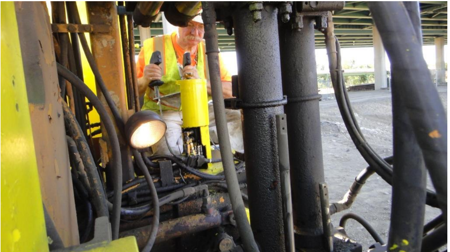
Mike H. lines up the spike over the hole in the tie-plate
