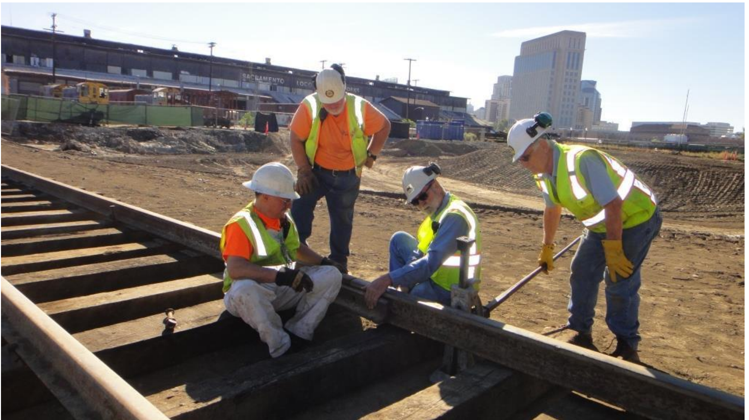
Mike H. and Alan line up joint bars while Mike W. adjusts the height of the rail with a track jack
